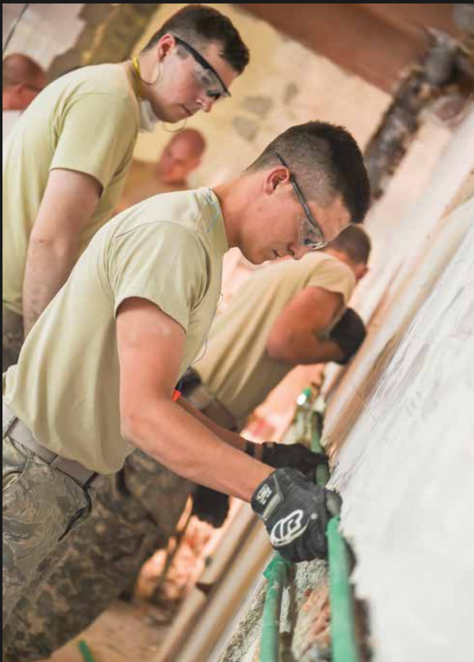
Airman First Class Derick Kvam of the 148th Civil Engineer Squadron out of Duluth, Minn. secures waterlines for kitchen appliances during a Humanitarian Civic Assistance project in Karlovac, Croatia on June 13, 2016. (Courtesy Photo)
